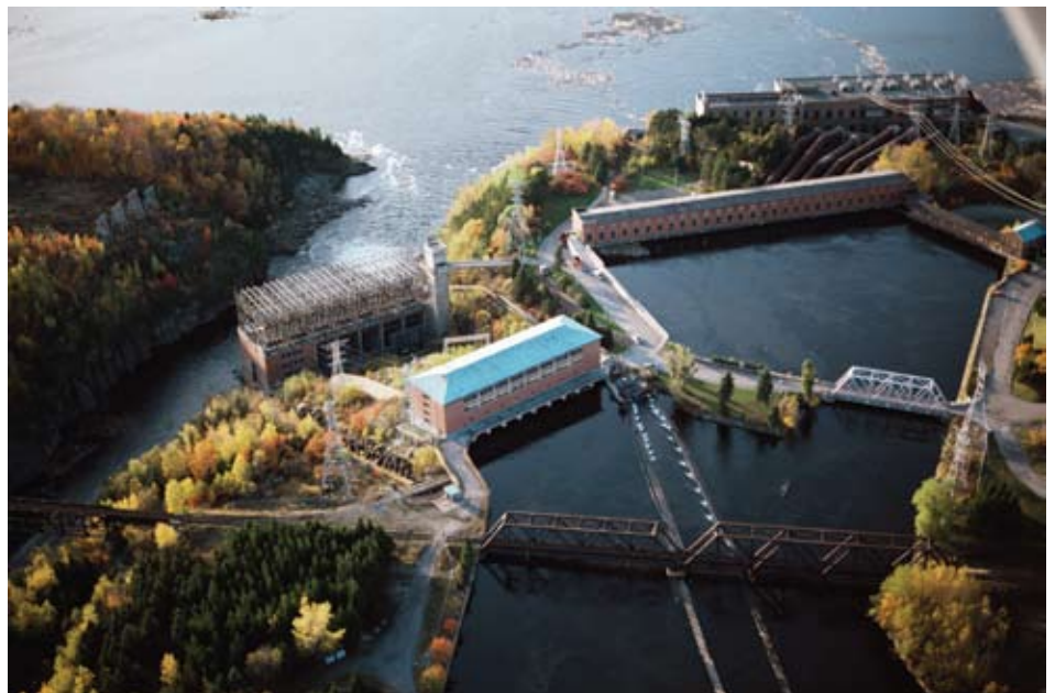
Aerial view of water impoundment in Canada (Jupiterimages)
